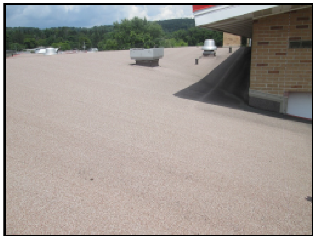
(C) EXISTING PHOTO - MAIN ROOF III
