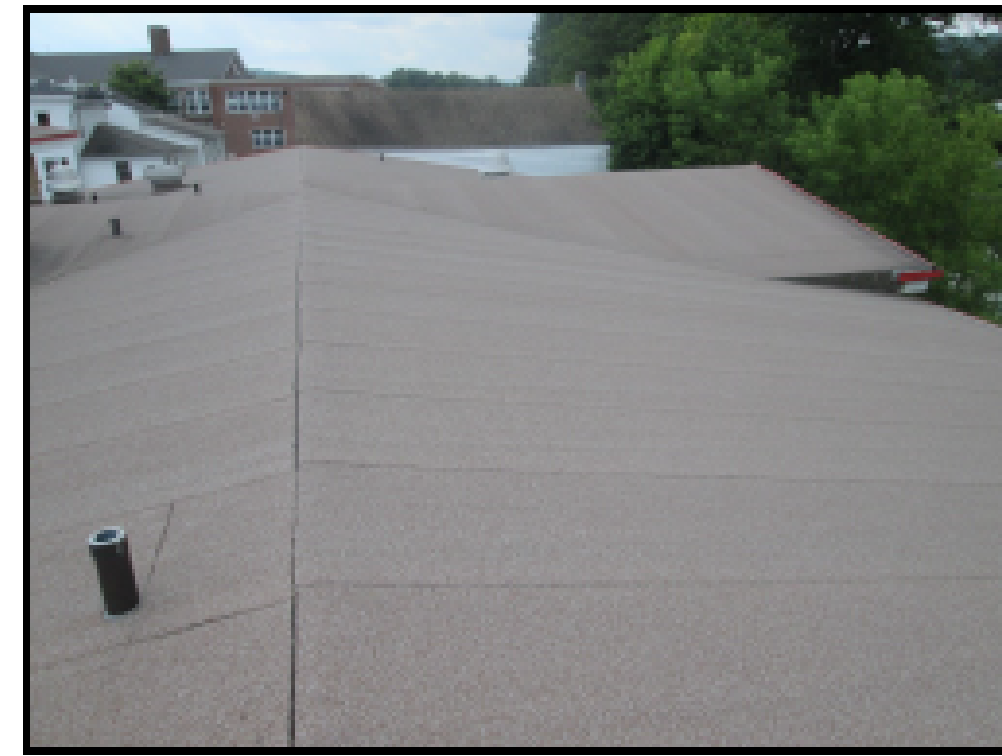
(A) EXISTING PHOTO - MAIN ROOF I
