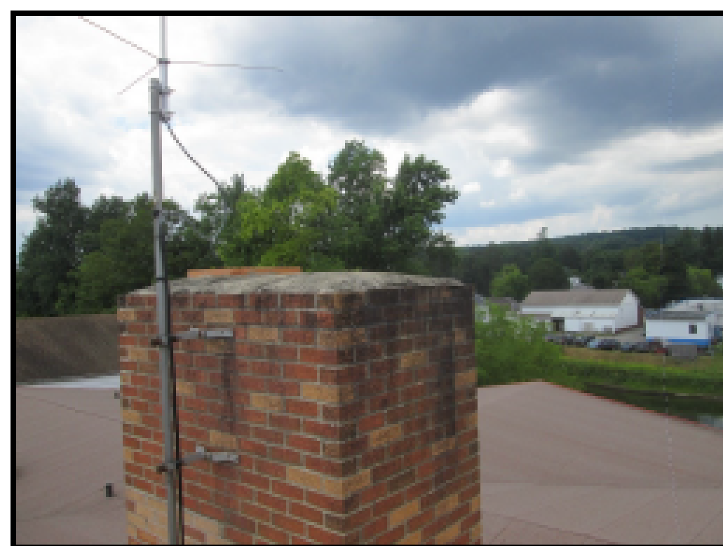
G EXISTING PHOTO - CHIMNEY
