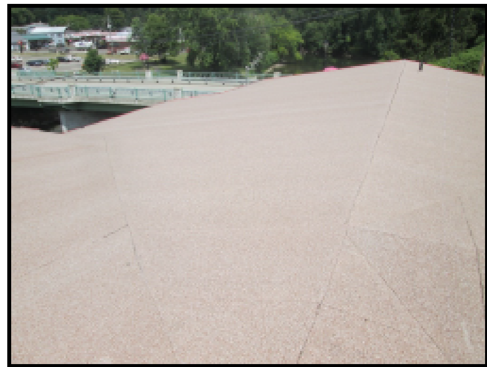
(B) EXISTING PHOTO - MAIN ROOF II
